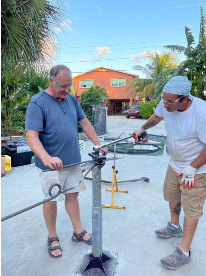
Figure 17. Dr. Steve Gittings and Peter Angeloti, bending rebar for frame. Angle and distance of each rebar bend was adjusted and finalized during the building process to create a final design template for future replication.
