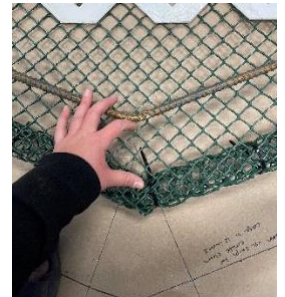
Figure 17. Using fingers to show about a 2" distance between the frame and the rolled plastic lattice.
