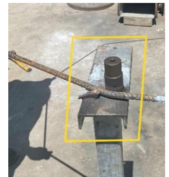
Figure 3. One of two 152.5-degree bends being bent on bending jig.
