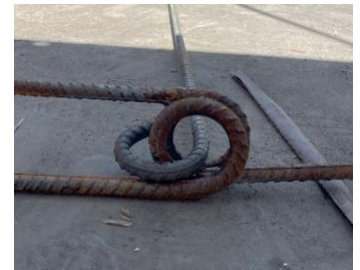
Figure 2. Deflector loop hinge, showing a 360-degree bend, used for a curved deflector (Step 8b). Outside loop is the deflector loop.
