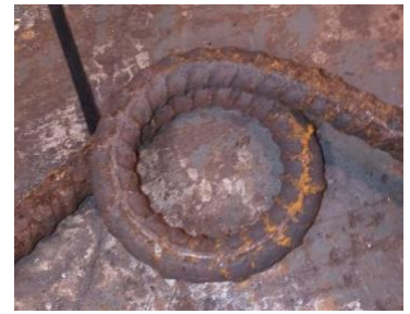
Figure 1. Deflector loop hinge, showing a 405-degree bend, used for a straight deflector (Step 8c).
