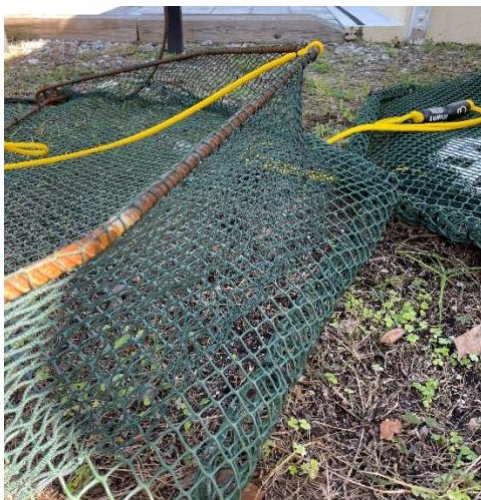
Figure 21. Finished installed netting between trap frame and hard plastic lattice. There should be minimal gaps between the netting, frame, and hard plastic lattice.
