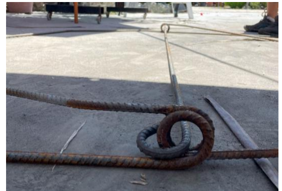
Figure 6. A different view of the same frames from Figure 5. End loop hinge with axle inserted through it and deflector hinge (closest loop), and loop on the end of axle connecting the two frames. The other end of the frame can also be seen from this view.
